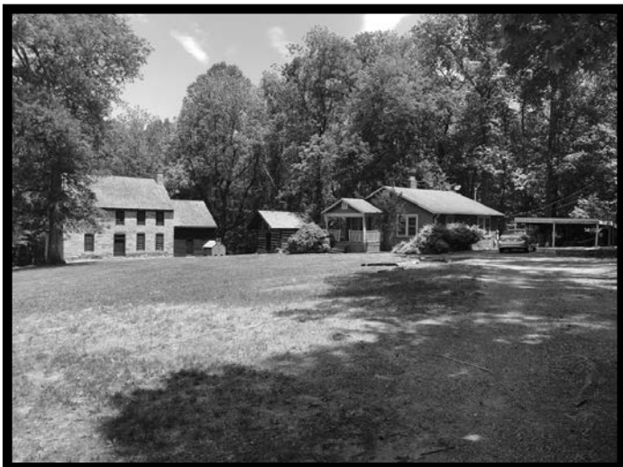
Before house and tree removal project
